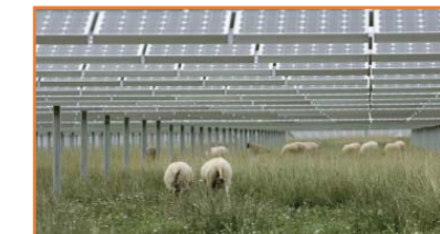
Farm solar generation system
